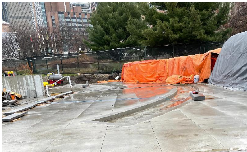
Construction on the memorial in December.
