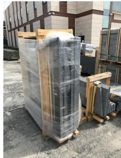
Construction is progressing.
